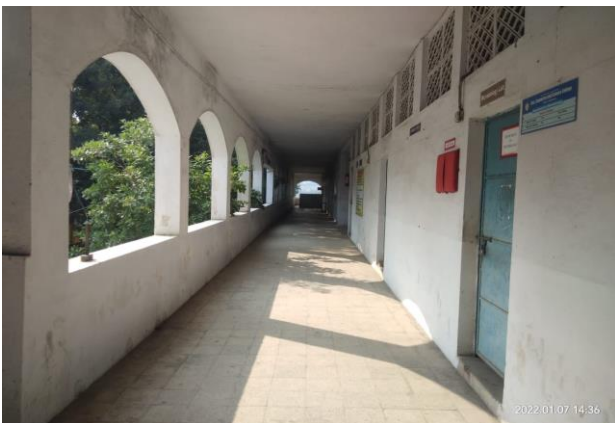
First Floor View
