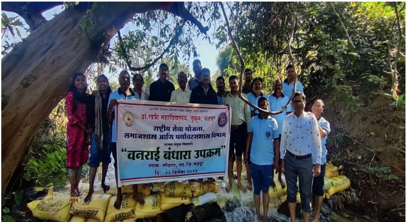
Fig- Construction of "Vanrai Bandhara" by NSS Unit
